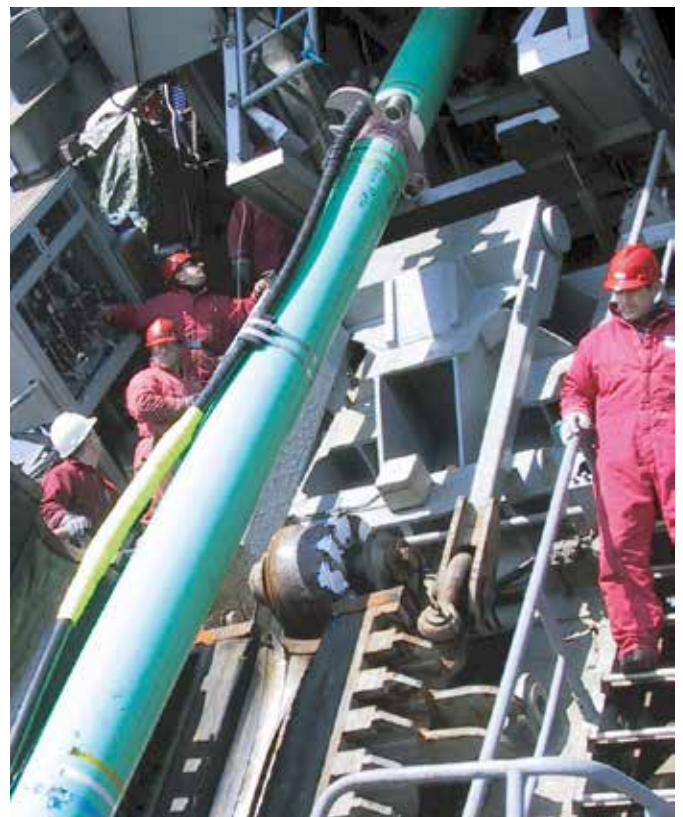
DEH cable installed with reel laying method
